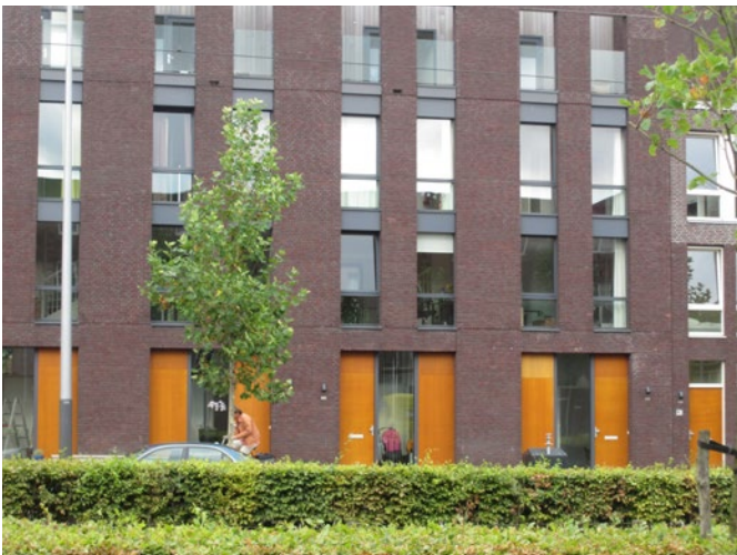
Example of a park edge frontage
