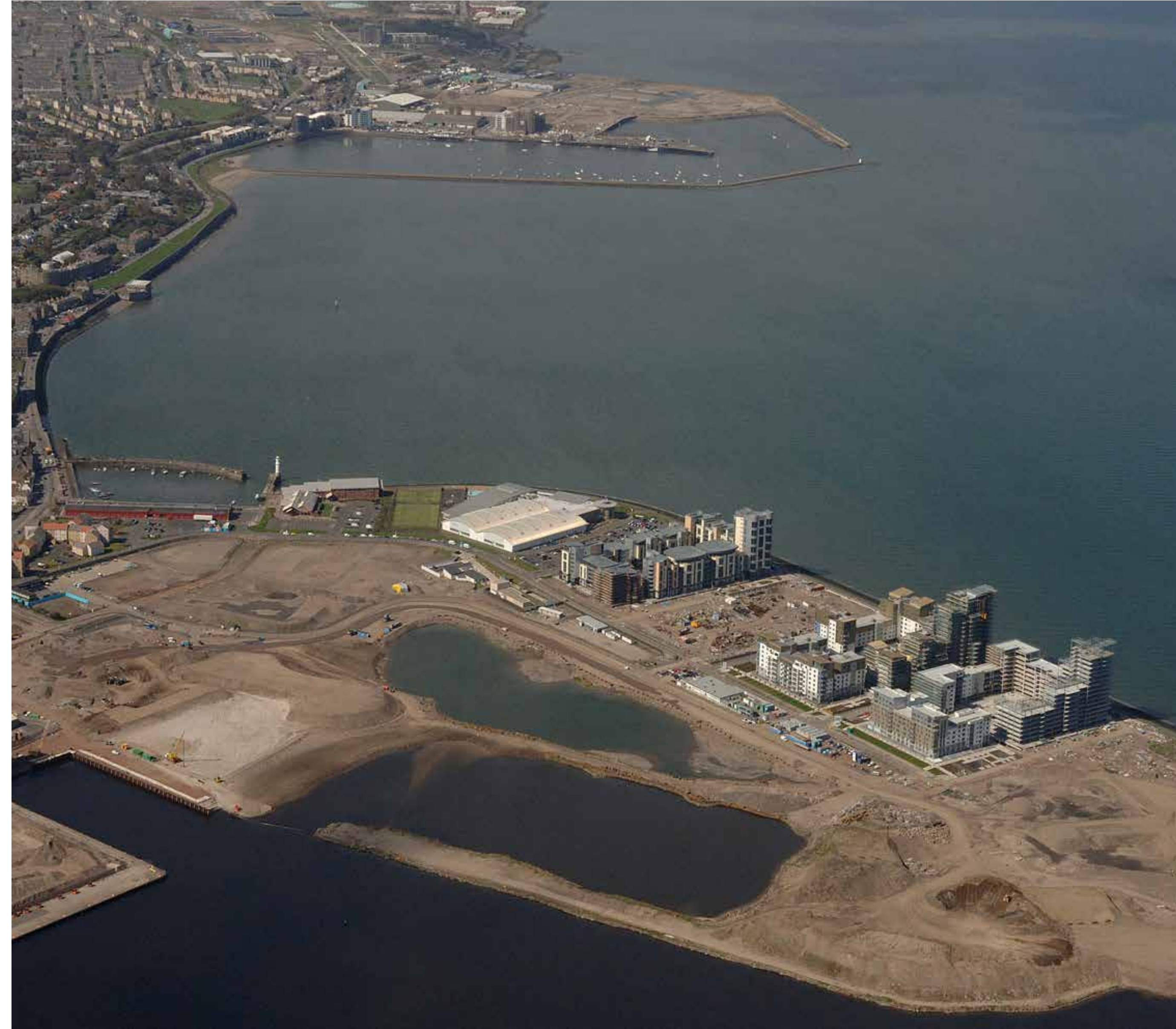
The site in 1990's during reclamation
